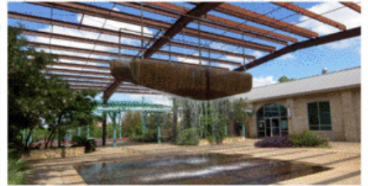
3601 South Congress- Existing Buildings
