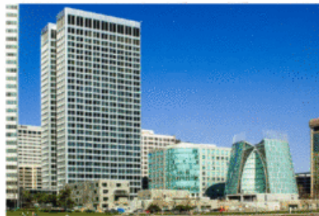
1 Kaiser Plaza – Existing Building
