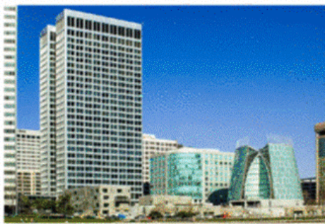
1 Kaiser Plaza – Existing Building
