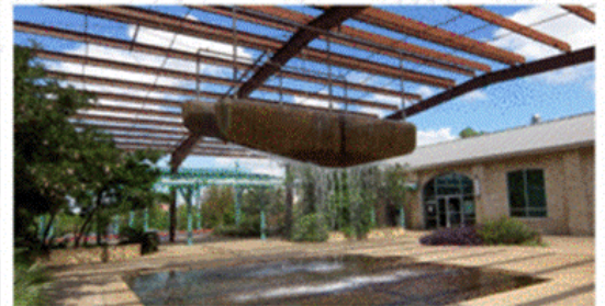
3601 South Congress- Existing Buildings
