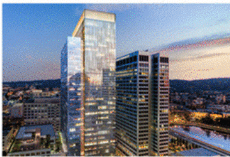
2 Kaiser Plaza (Beacon Tower), Oakland, CA
