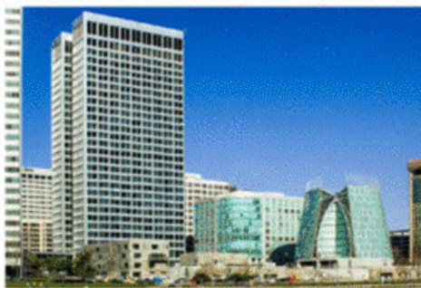
1 Kaiser Plaza – Existing Building
